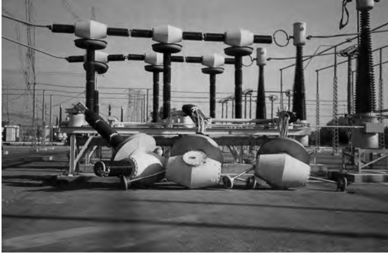
FIGURE 13.1 500kV live tank circuit breaker. (Photo courtesy of E. Matsuda, Copyright 1989–2011 Pacific Gas and Electric Company, Oakland, CA. All rights reserved.)
