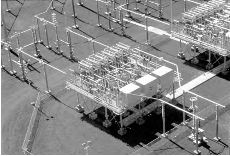
FIGURE 5.27 Aerial view of BPA's Slatt, Oregon, 500 kV TCSC. (Photo courtesy of GE, Fairfield, CT.)
