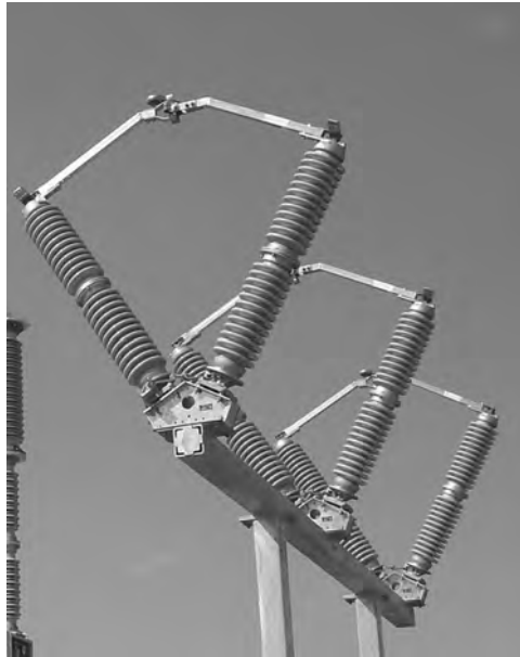
FIGURE 4.15 Center break “Vee” disconnect switch.
