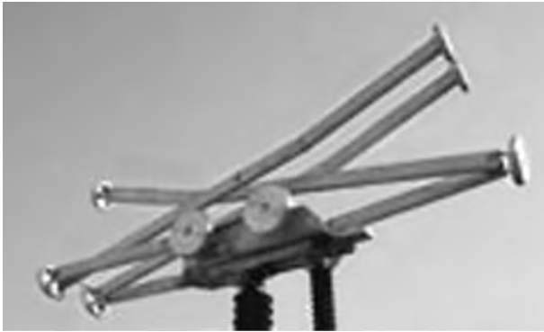
FIGURE 4.17 Vertical reach (pantograph) disconnect switch.
