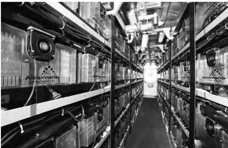
EXHIBIT 21.8 Mobile utility battery storage. (Courtesy of Altairnano, Reno, NV.)
