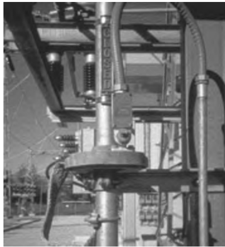
FIGURE 4.1 Mechanical cam-action type interlock.
