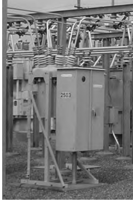
FIGURE 4.38 Single-tank bulk oil circuit breaker.
