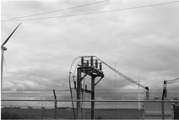
FIGURE 4.16 Single side break disconnect switch.
