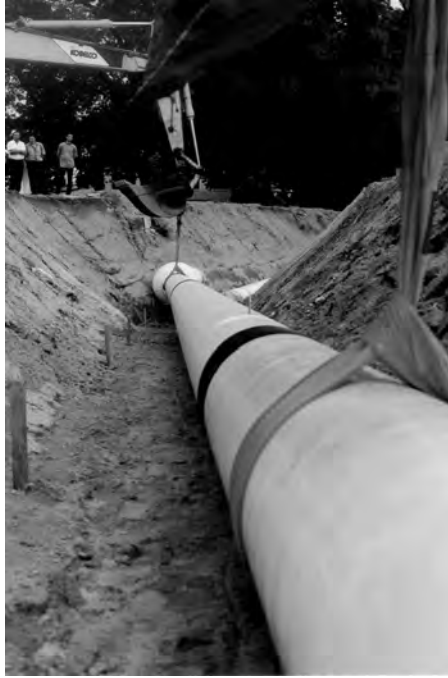
FIGURE 18.5 Laying the GIL into the soil. (Courtesy of Siemens AG, Erlangen, Germany.)
