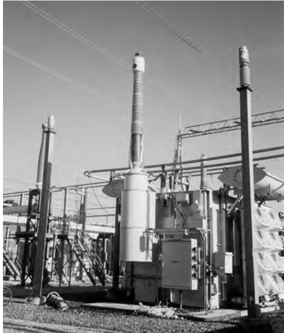
FIGURE 13.3 Porcelain bushing. (Photo courtesy of E. Matsuda, Copyright 1996–2011 Pacific Gas and Electric Company, Oakland, CA. All rights reserved.)
