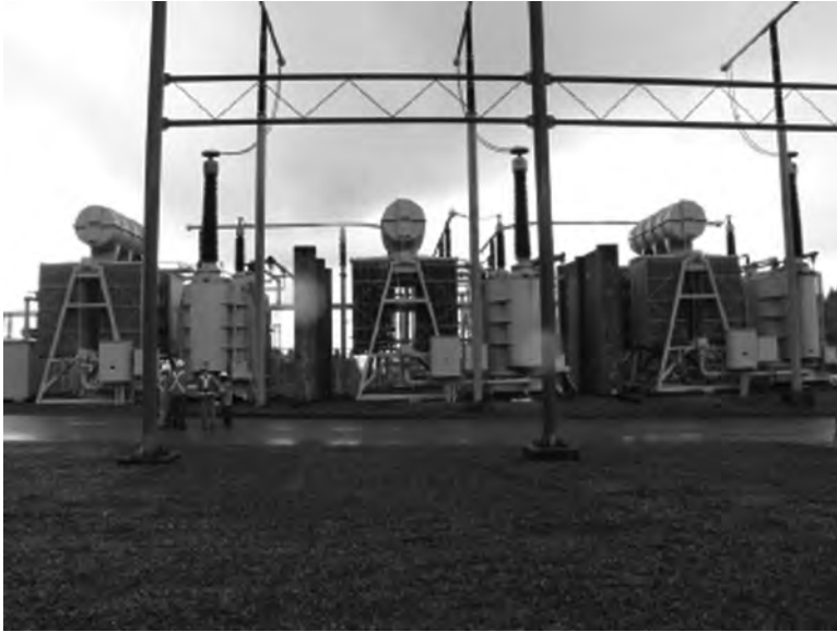
FIGURE 14.4 Fire barriers between individual single-phase transformers that are not high enough to protect the 230kV bushings on adjacent transformers.
