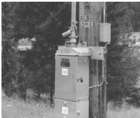
FIGURE 4.7 Stored energy motor operator for disconnect switch.
