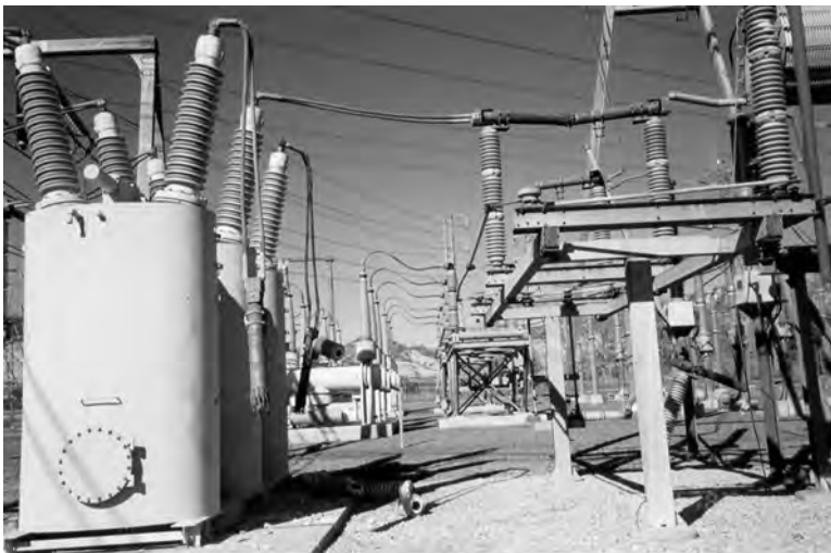
FIGURE 13.4 230 kV circuit breaker and air disconnect switch. (Photo courtesy of E. Matsuda, Copyright 1996–2011 Pacific Gas and Electric Company, Oakland, CA. All rights reserved.)
