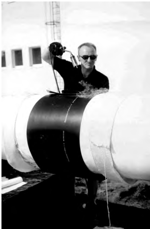
FIGURE 18.30 On-site corrosion protection of the welding area—shrinking method. (Courtesy of Siemens AG, Erlangen, Germany.)
