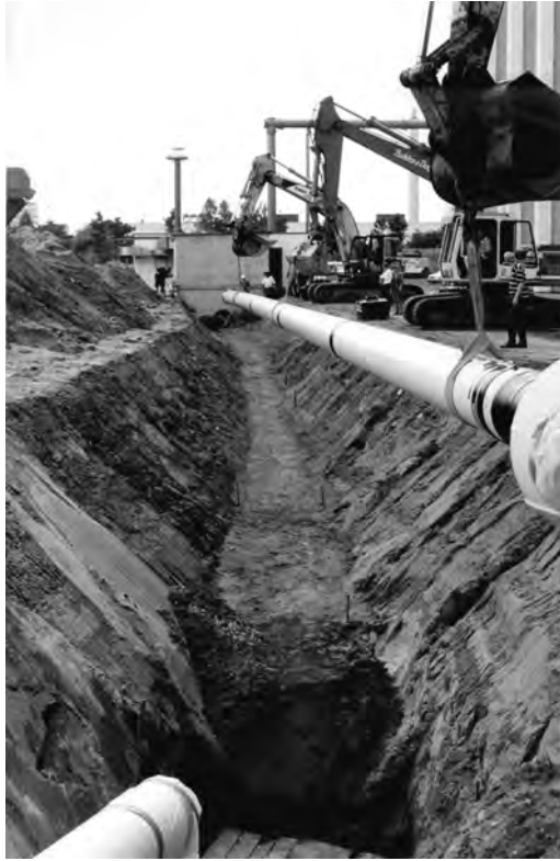
FIGURE 18.20 Trench of 55-m-long section during laying and view into the trench. (Courtesy of Siemens AG, Erlangen, Germany.)
