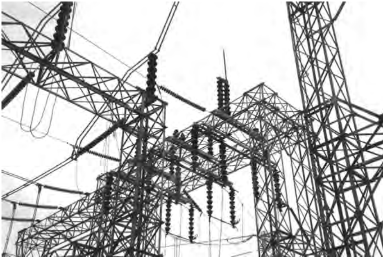
FIGURE 13.2 230kV air disconnect switch. (Photo courtesy of E. Matsuda, Copyright 1989–2011 Pacific Gas and Electric Company, Oakland, CA. All rights reserved.)
