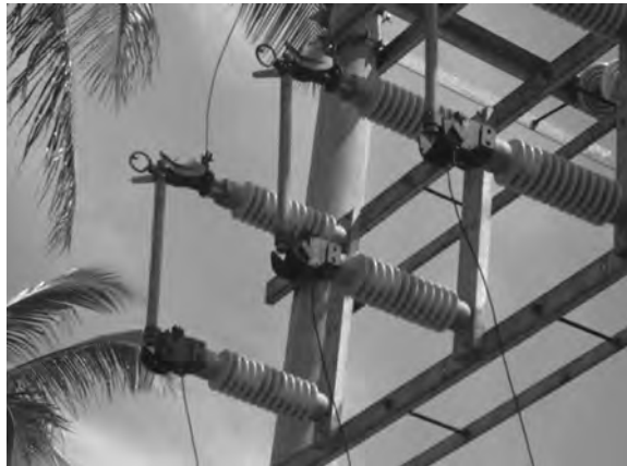
FIGURE 4.32 Vertically mounted power fuses.
