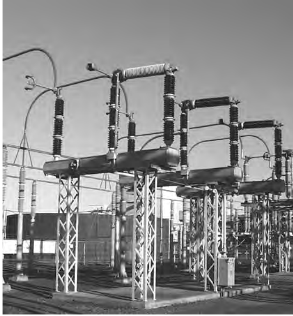
FIGURE 4.33 Multiple interrupter gap per phase circuit switcher.
