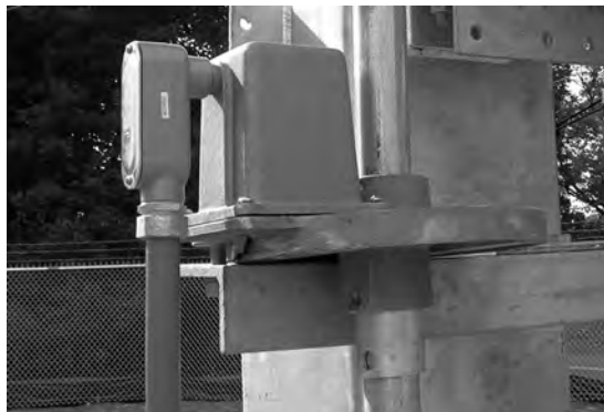
FIGURE 4.3 Solenoid type interlock.
