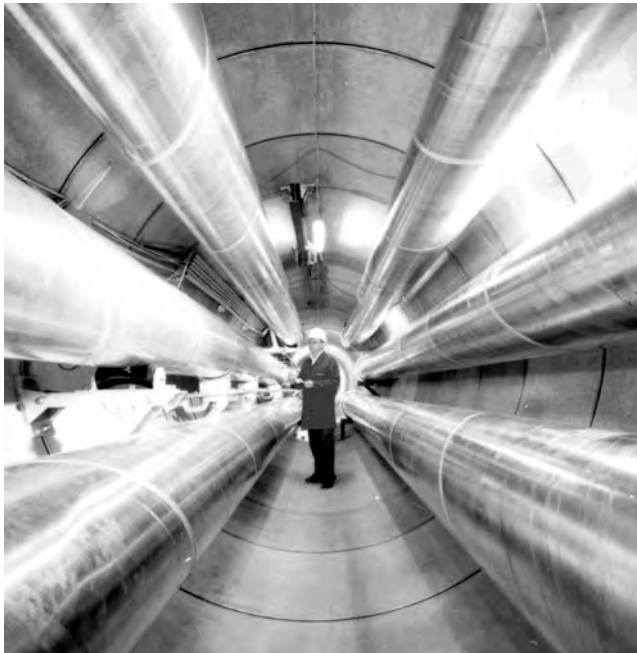
FIGURE 18.7 View into the tunnel. (Courtesy of Siemens AG, Erlangen, Germany.)
