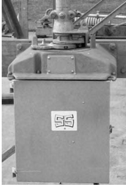
FIGURE 4.6 Motor operator for disconnect switch.
