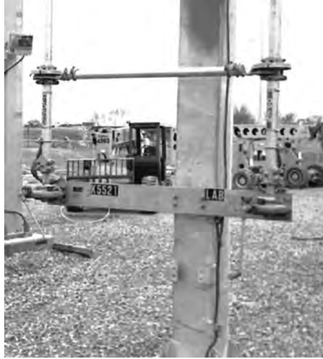
FIGURE 4.1 Mechanical cam-action type interlock.
