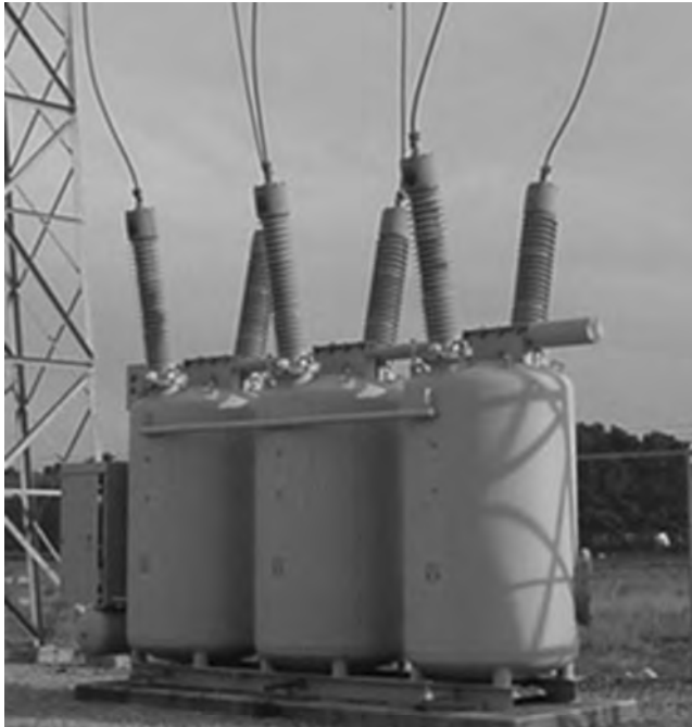
FIGURE 4.39 Three-tank bulk oil circuit breaker.
