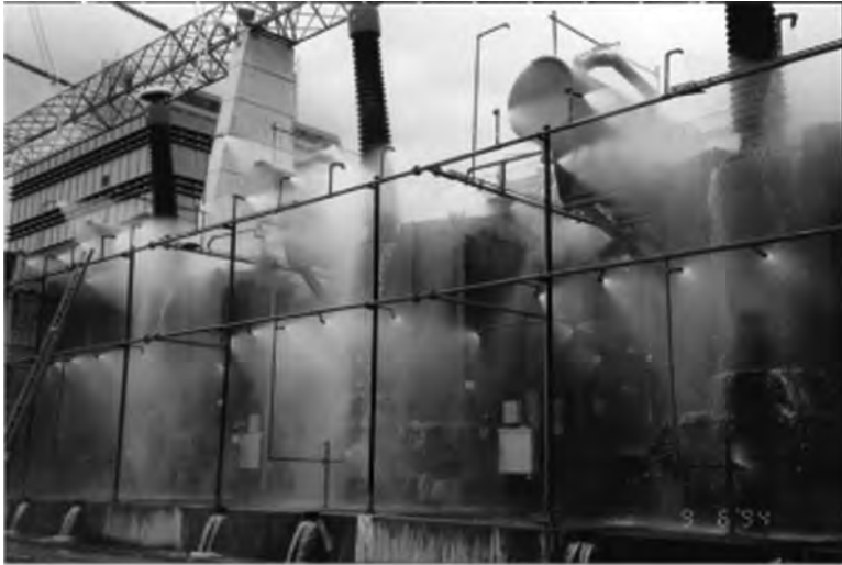
FIGURE 14.5 Transformer deluge system in operation.
