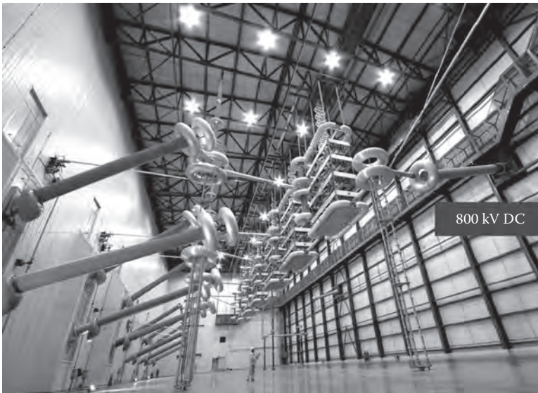
FIGURE 5.12 800 kV UHV DC Yunnan–Guangdong—view of the bipolar valve halls with two 400kV systems in series to build 800kV.
