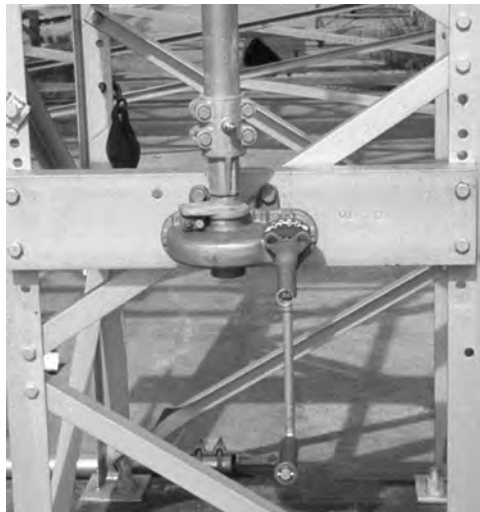
FIGURE 4.5 Gear crank operator for disconnect switch.
