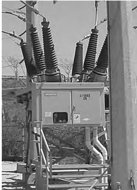
FIGURE 4.41 SF 6 gas dead tank circuit breaker.
