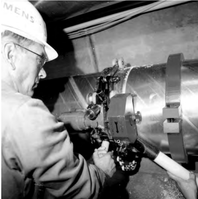
FIGURE 18.18 Cutting the enclosure pipe with a saw. (Courtesy of Siemens AG, Erlangen, Germany.)
