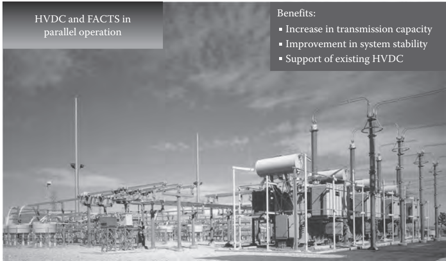
FIGURE 5.22 FACTS shunt compensation for system upgrade: 2 SVCs Mead-Adelanto, 500 kV, each at 388 MVar cap.—United States, 1995.
