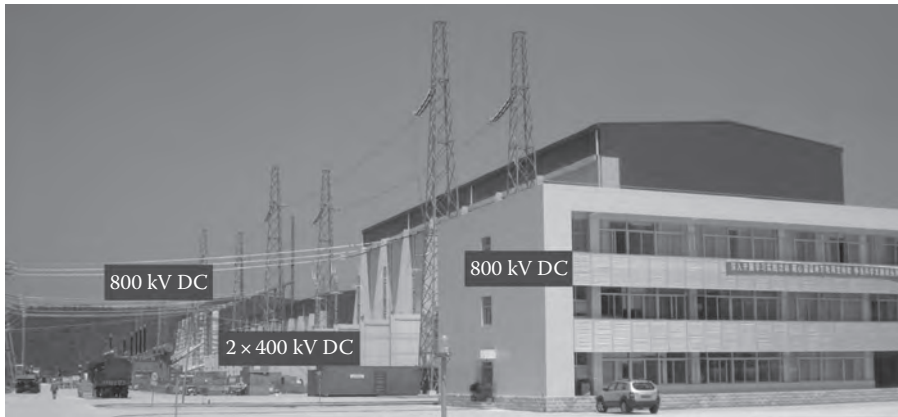
FIGURE 5.14 China—comparison of UHV AC (1000kV pilot project, left side) (Photo courtesy of State Grid, Beijing, China.) and UHV DC lines (800kV, right side). (Photo courtesy of Siemens AG, Erlangen, Germany.)
