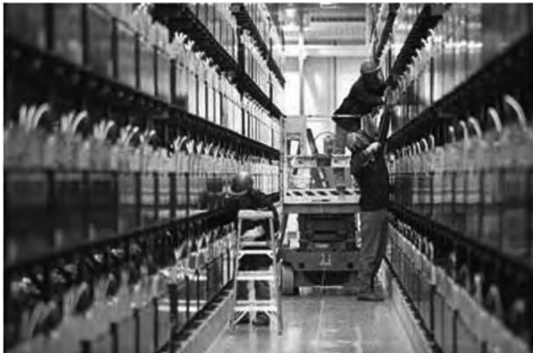
EXHIBIT 21.7 Nickel-metal hydride battery system. (Courtesy of Pennwell, Tulsa, OK.)
