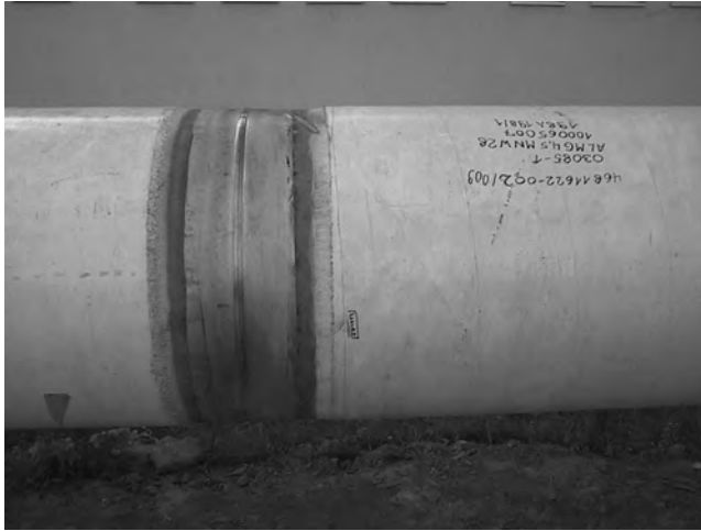
FIGURE 18.29 GIL with passive corrosion protection. (Courtesy of Siemens AG, Erlangen, Germany.)
