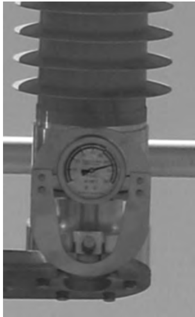
FIGURE 4.29 SF 6 interrupter's pressure indicator.
