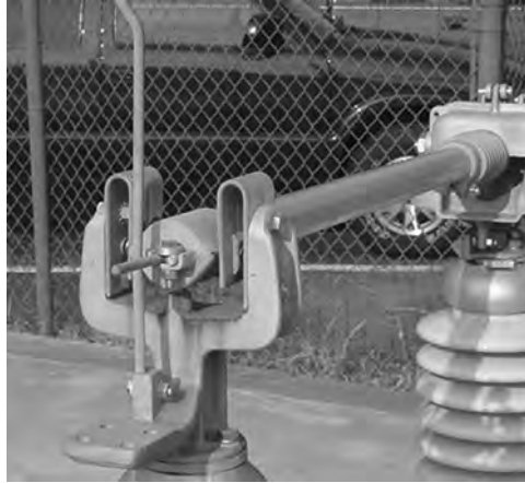
FIGURE 4.25 Arcing horns on a vertical break switch.
