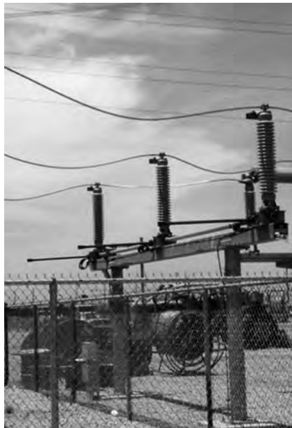
FIGURE 4.17 Vertical reach (pantograph) disconnect switch.
