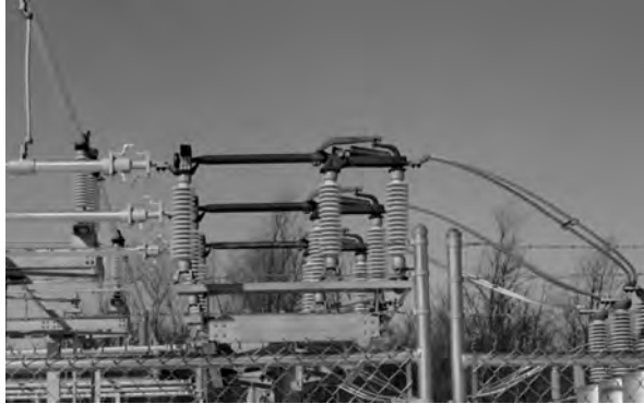
FIGURE 4.8 Horizontally upright mounted disconnect switch.
