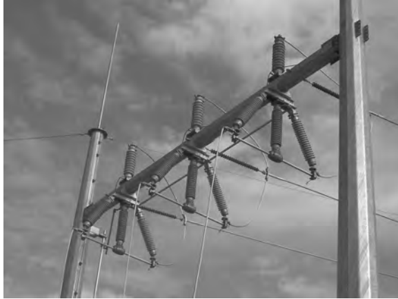
FIGURE 4.10 Under hung mounted disconnect switch.
