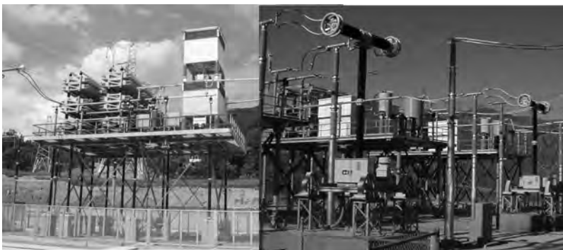
FIGURE 5.28 FSC: fixed series compensation, Fengjie, China, 500 kV, 2 \times 610 MVar and TPSCs Vincent, Midway, and El Dorado/USA, seven systems at 500 kV.
