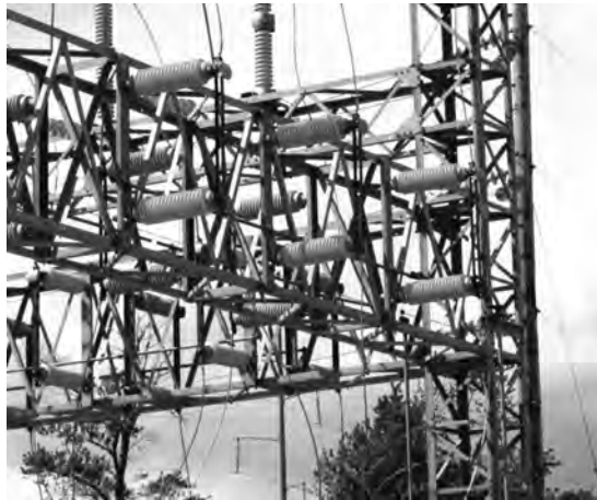
FIGURE 4.9 Vertically mounted disconnect switch.
