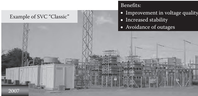
FIGURE 5.24 SVC São Luis, ELETRONORTE, Brazil: TCR, TSC/FC, 230 kV, 150 MVar cap./100 MVar ind.
