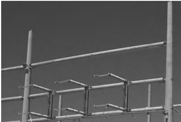
FIGURE 4.23 Vertically mounted center break disconnect switch.
