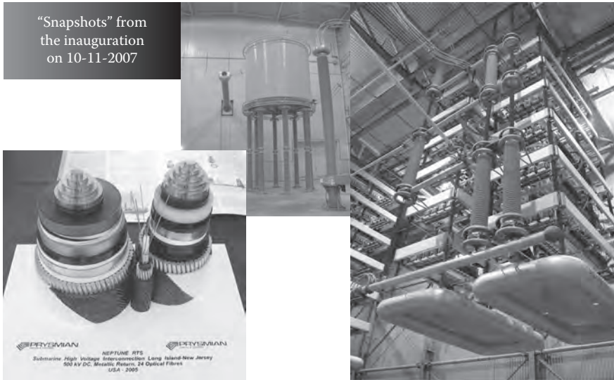
FIGURE 5.6 Neptune HVDC—a view of Station Duffy Avenue inside: the cable, indoor smoothing reactor, and thyristor converter.
