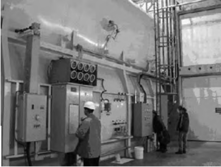
FIGURE 14.1 Shows large distribution transformer in an explosion containment tank inerted with nitrogen.
