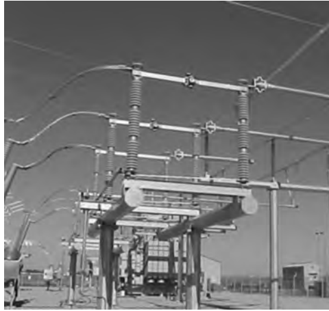
FIGURE 4.14 Center break disconnect switch.
