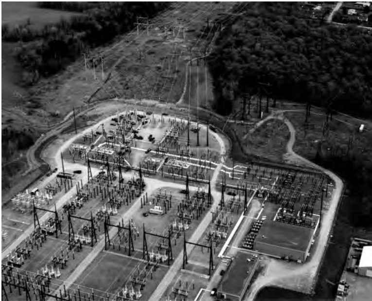
FIGURE 5.36 CSC at NYPA's 345 kV Marcy, New York.
